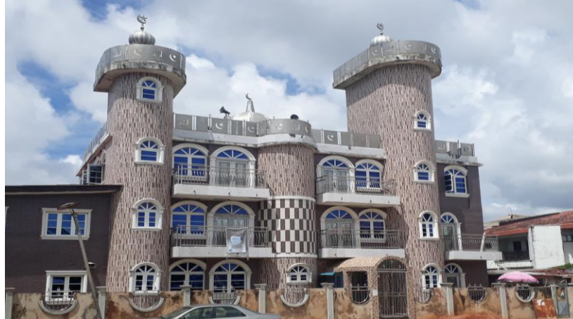
Fig 1: A front view of the renovated FTMC Central Mosque, FESTAC-Town, Lagos
